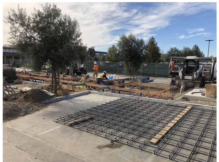
Workers prepare conduits and wiring in preparation for a concrete pour.
