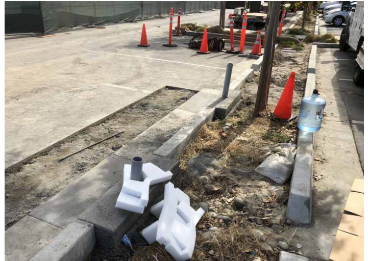
Plastic wiring conduits emerge at the curb edge indicating where Tesla Supercharger dispensers will be installed.
