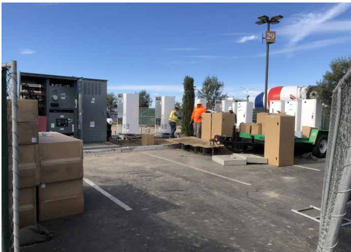
A cluster of white Tesla charger cabinets is installed to the right of a large gray electrical switchboard.
