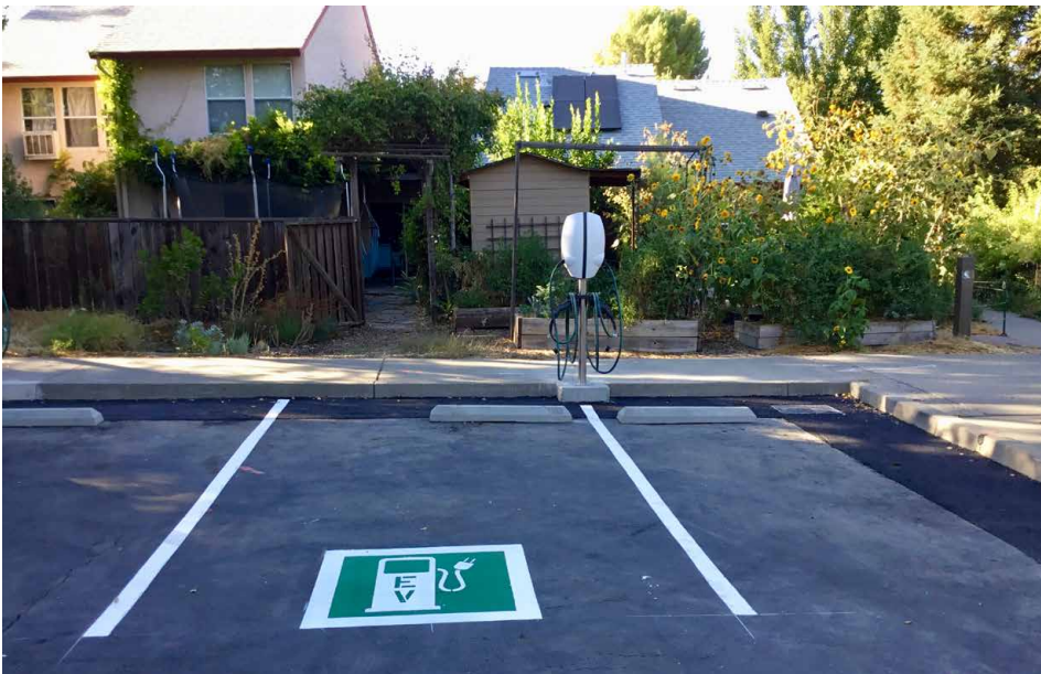
This dual pedestal can really only provide two stalls with EV charging power. It could be an example of what NOT to do. If this post were centered in the marked stall – the cables might stretch to cover three parking stalls.
