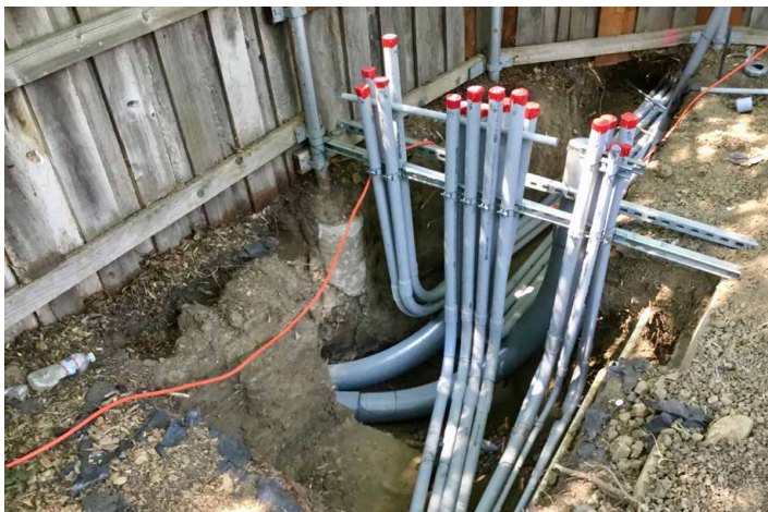
Each small conduit is for a charging station (EVSE). The larger conduit is for the on-site step-down transformer which gets fed from a higher voltage transformer located upstream (possibly fed from overhead wires).
