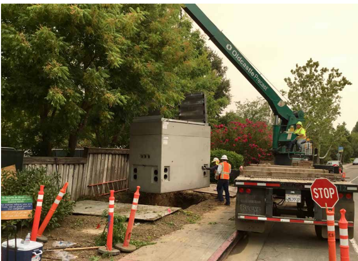
Underground vault installation begins.
