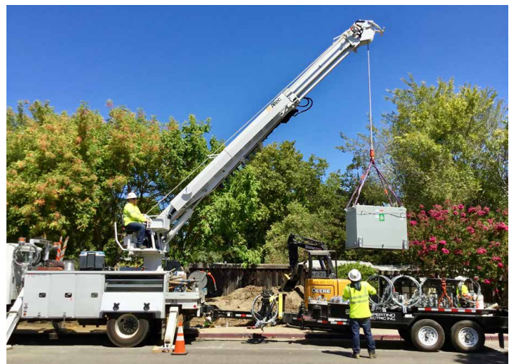
Lifting of the several hundred KVA (and pounds!) transformer from the truck. Such units typically power a half dozen residences.
