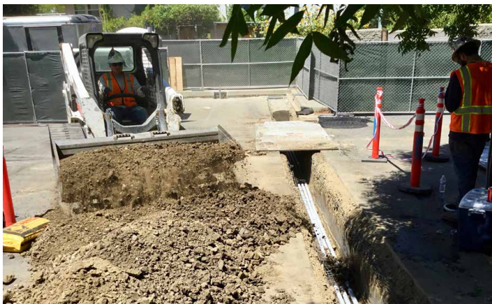
Plastic conduit is placed to accommodate the feeders to the EVSE. With trenching complete, backfilling begins.
