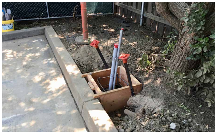
Conduit in place ready for concrete. The trench has been backfilled.
