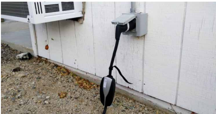
Jesla mobile charge cable and NEMA 14-50 adapter can provide up to 40 amps continuous at 240 volts.
