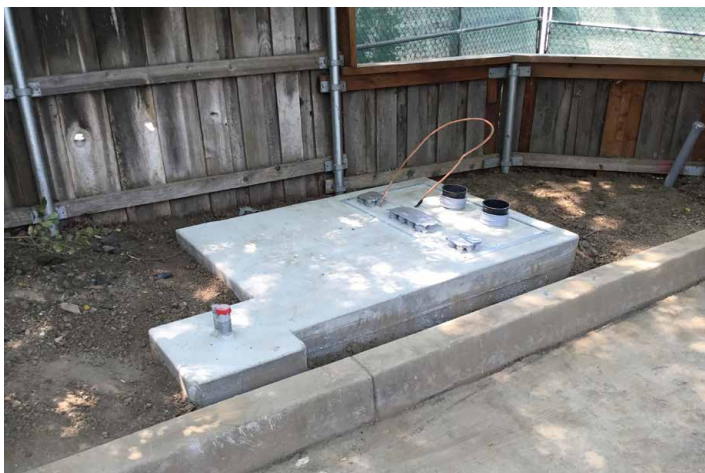
Transformer pad with conduit to vault plus one pedestal base.
