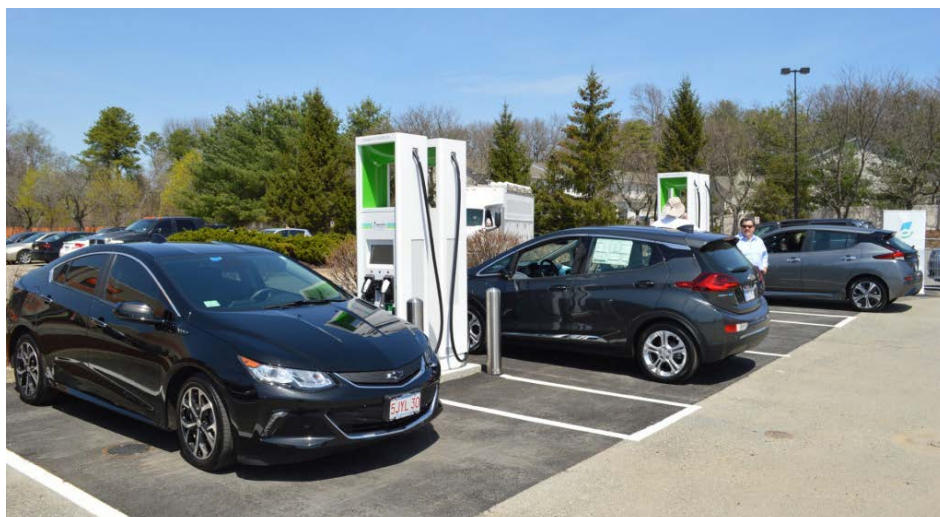
Electrify America 350 kw chargers at Home Depot in Chicopee, MA
