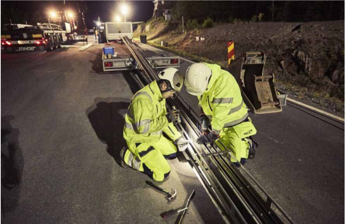
Workers install the electric rail underneath the road.
